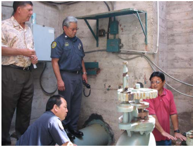
KEEPING THE WATER SAFE. BWS employees joined with members of the Honolulu Police and Fire Departments, and Civil Defense in an emergency preparedness exercise.
