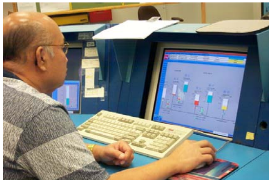
WATCHFUL EYE. The Control Center staff monitored the BWS water system around-the-clock through the Supervisory Control and Data Acquisition (SCADA) system.
