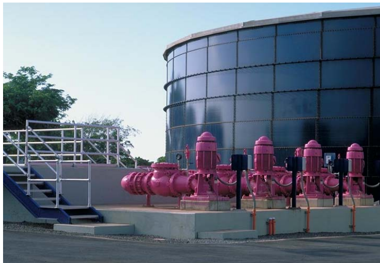
Honouliuli Water Recycling Facility. This BWS facility is designed to generate 12 million gallons of recycled water per day for irrigation and industrial uses.
