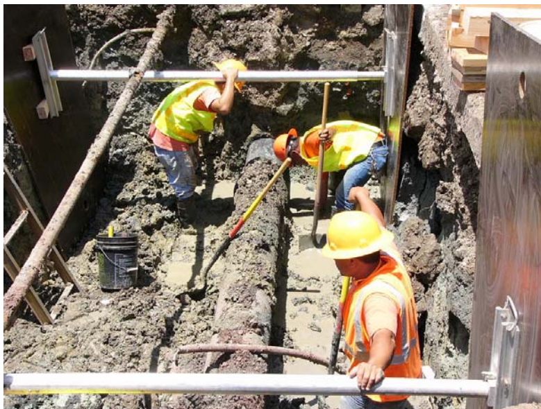
May 2007 Liliha Street main break. BWS crews often work in muddy trenches under bad weather conditions, day and night, to quickly restore water service to customers.
