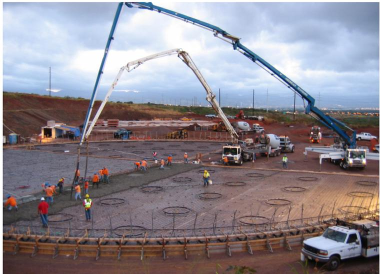
**Reservoir Construction.** Crews work on the foundation of the new Honouliuli 228 Reservoir No. 3.
