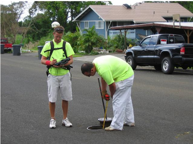
**Contractor's help map BWS assets using Global Positioning System technology**
