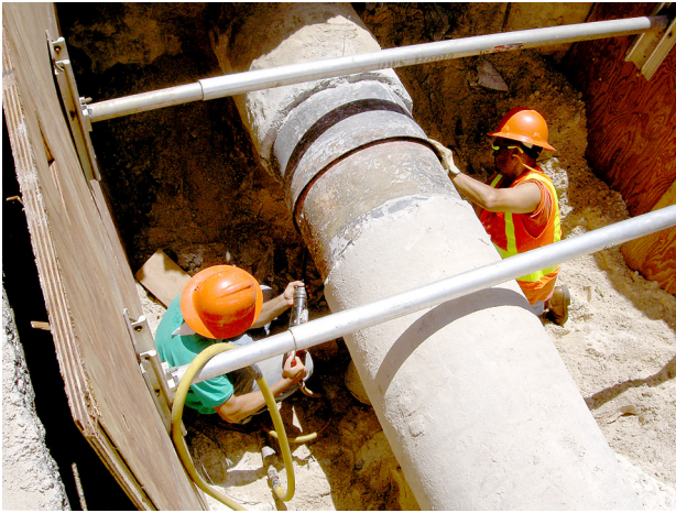
Water Main Breaks. BWS Field Operations crews respond to water main breaks to minimize water loss and to restore water service as quickly as possible.
