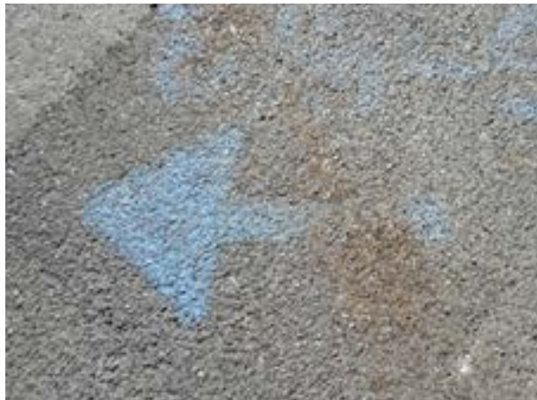
Markings to Identify Meter Locations
