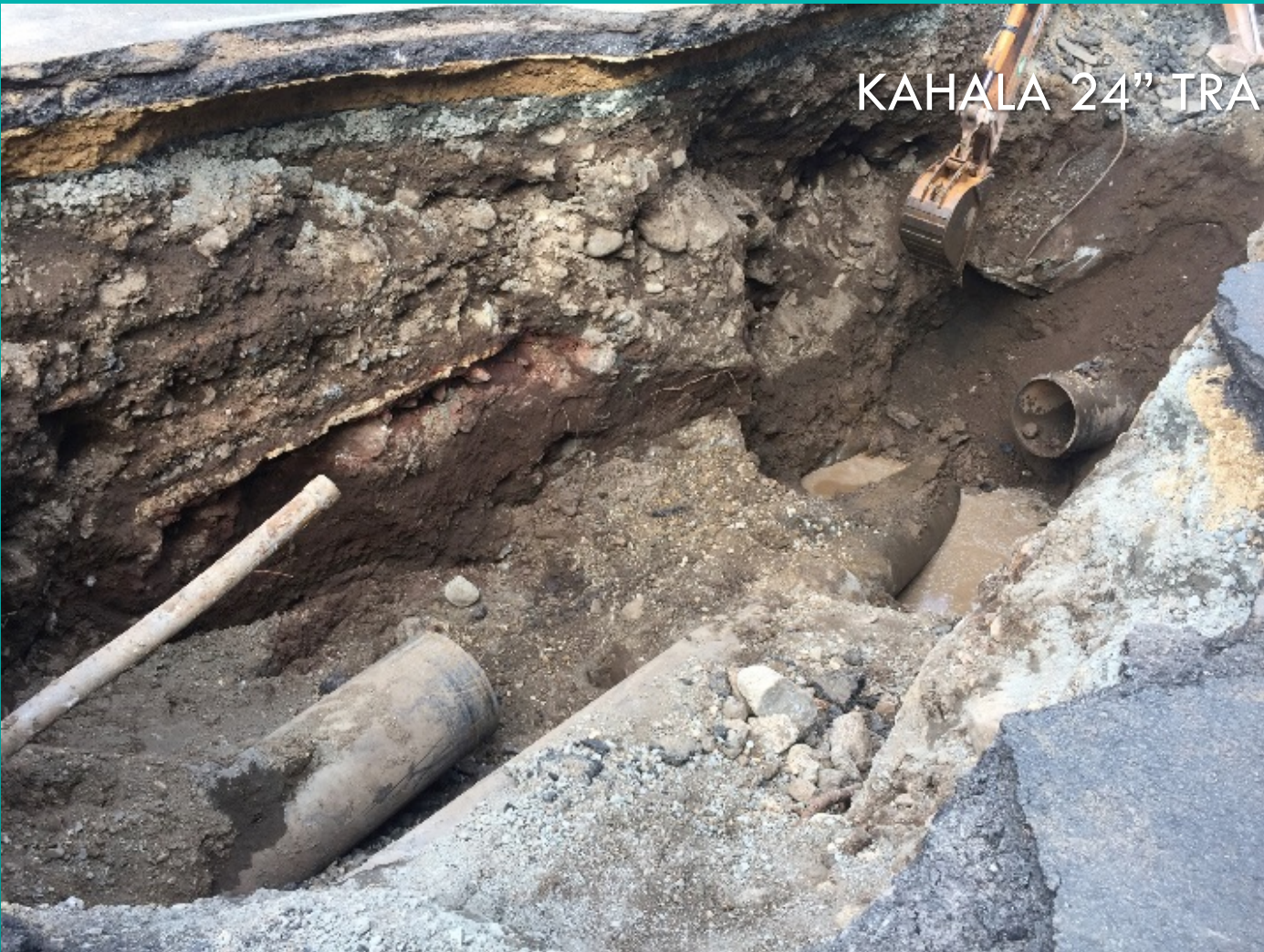
Abandoned Main on Top, Live Main Underneath
