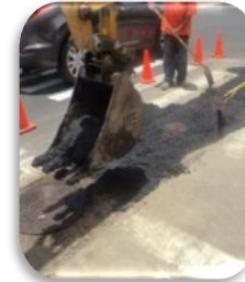
Crews install temporary asphalt to fill the trench until final restoration of the road.
