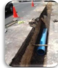
Base course and backfill over installed pipe.
