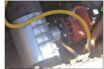
Valves and pipes are pressure tested before final connections.
