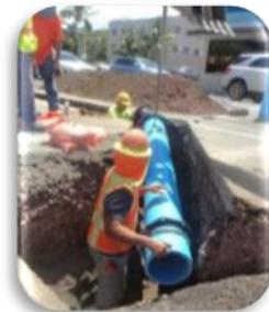
Crews carefully install PVC pipe and secure it tightly.
