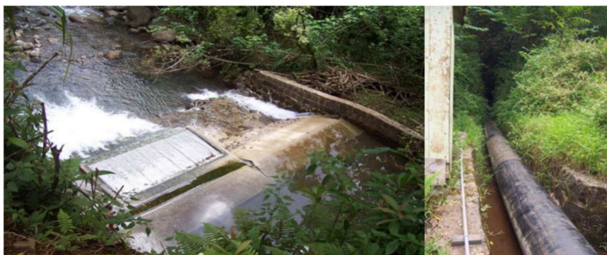
Figure 1-7: Punalu'u Stream Diversion and Piped Ditch
