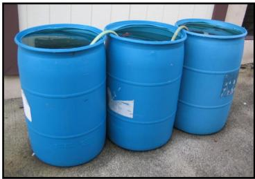
These rain barrels have an overflow near the top. The hose for the overflow can either be directed towards your yard or into another barrel.
