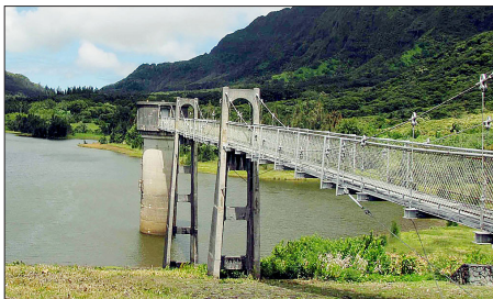
Nuuanu Reservoir No. 4 features a tower which contains three gates or valves which help regulate the water level.
