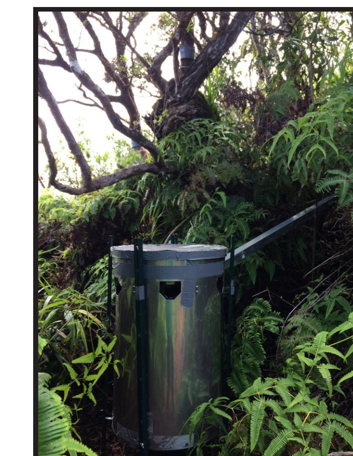
Throughfall Equipment: For each test plot, a total of three troughs lead to a fabricated tipping bucket (150 mL / tip) rain gauge. The gauge is nested in a stainless steel can, levelled and anchored to the ground for stability. Troughs were installed under trees typical of the test plots (species, diameter, height) in configurations that represented the average canopy and gap proportions and minimized overlap of throughfall collection between troughs.
