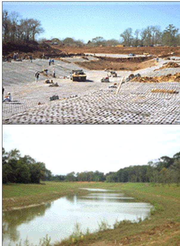
**Interlocking block design (above) allows for infiltration of stream water, vegetation growth, and erosion control (below)**
