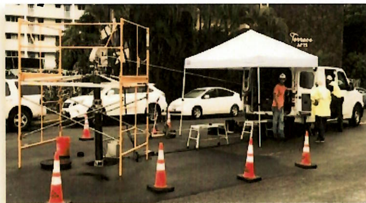
Advanced pipeline condition assessment requires traffic control, excavation, construction of a vault, tapping into water-filled pressurized pipe, and installation of a valve. The testing team tracks a probe inserted into the pipeline, propelled by the moving flow of water, up to a distance of 1/2 mile.
