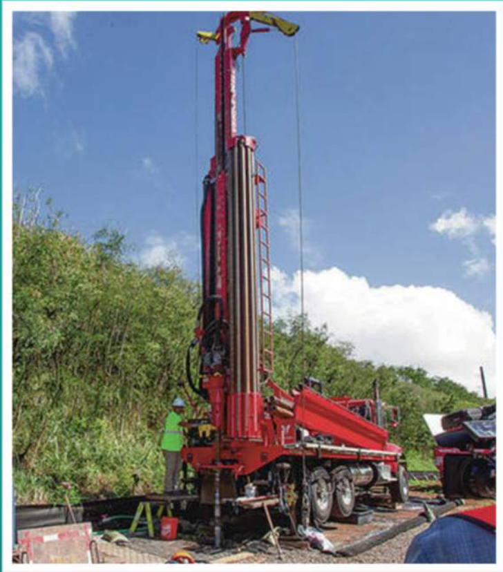
BWS Monitoring Well Installation, February 2024 Source: Honolulu Star-Advertiser
