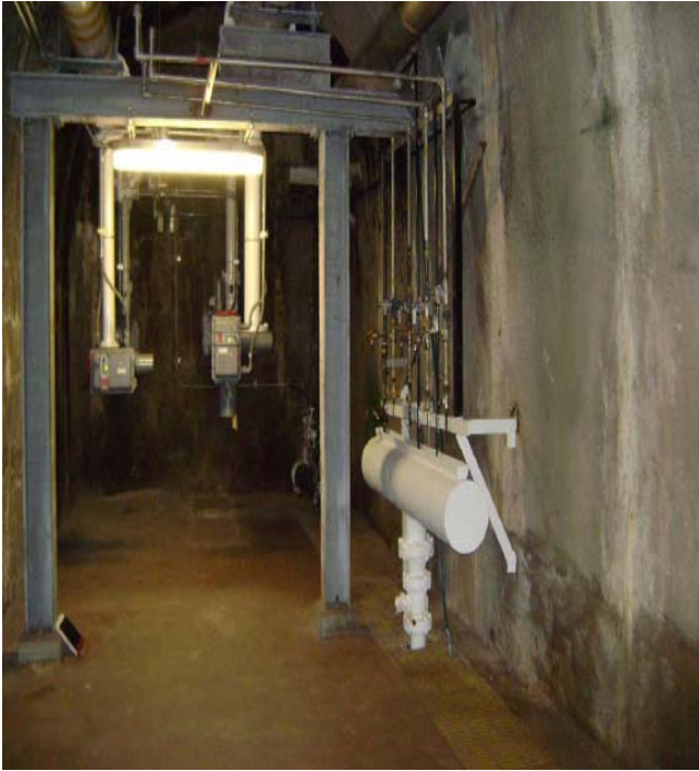
Figure 2: Typical Tank Bottom Access
