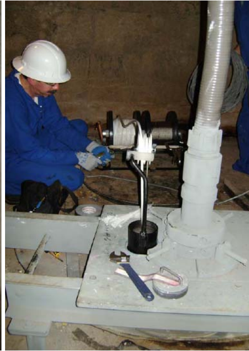
Figure 3: Typical Tank Top Access
