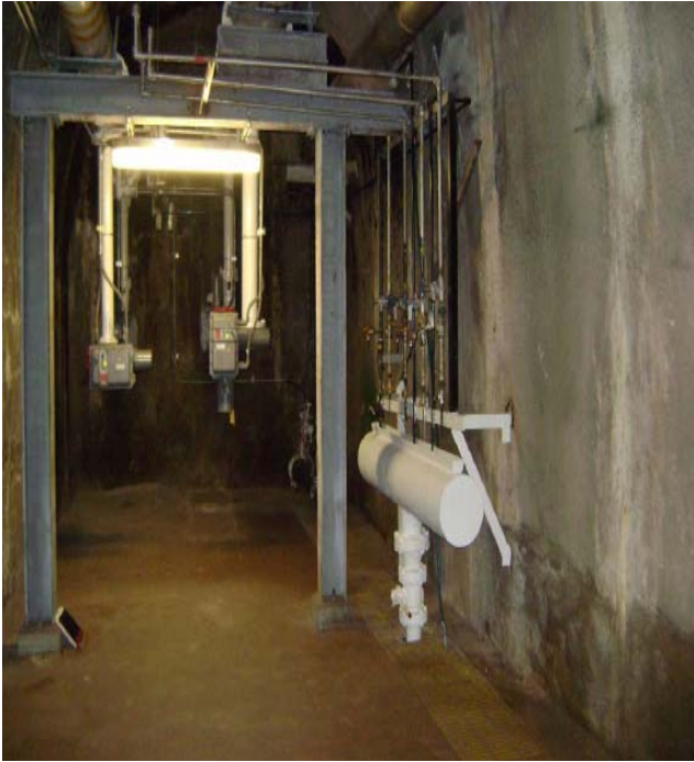
Figure 2: Typical Tank Bottom Access
