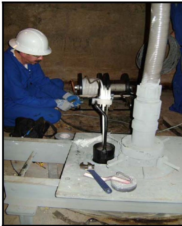
Figure 1-3: Typical Tank Top Access
