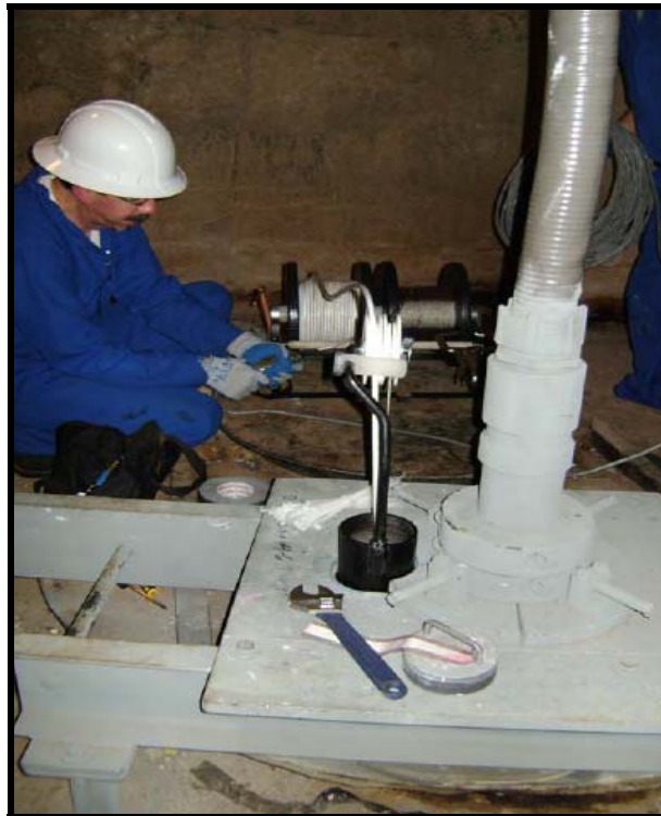
Figure 1-3: Typical Tank Top Access
