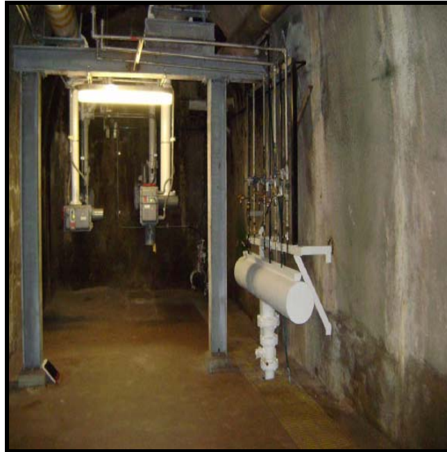
Figure 1-2: Typical Tank Bottom Access
