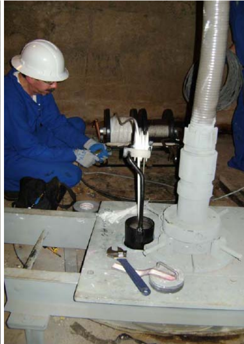
Figure 3: Typical Tank Top Access
