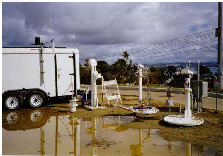
Figure 13. Tank 175 at the Point Loma Fuel Terminal.
