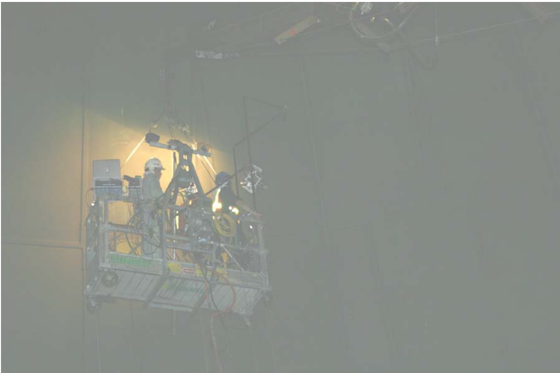
Inspection team #1 using the Viper LFET/U.T. Crawler on course C in Quadrant C of the Upper Dome.
