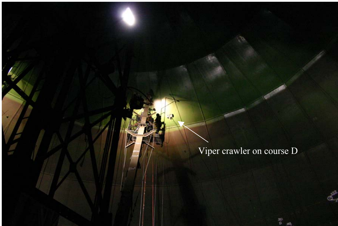
A view from the catwalk of the Viper Crawler performing an Ultrasonic Inspection of course D of the Upper Dome.
