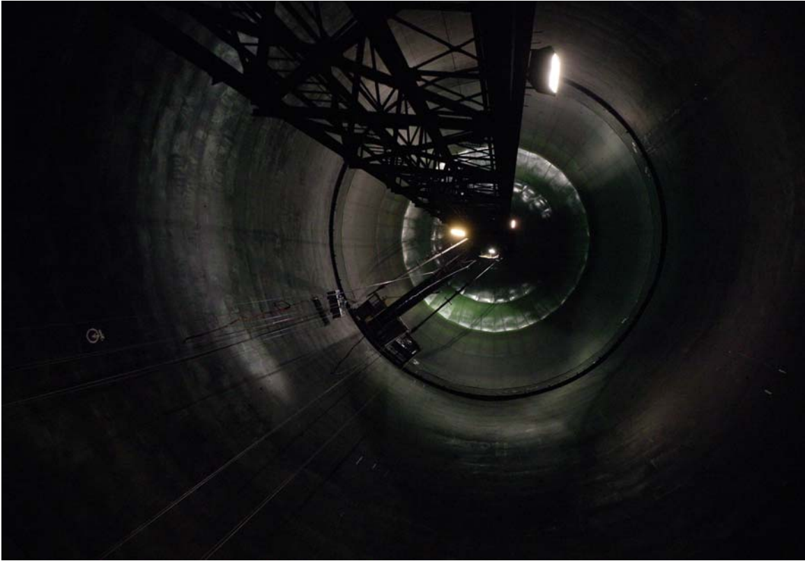
A view of tank #15 from the floor looking upward.
