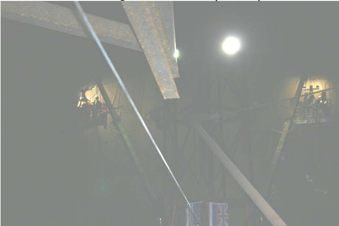
Both inspection crews in the Upper Dome during Viper LFET/U.T. Crawler work.
