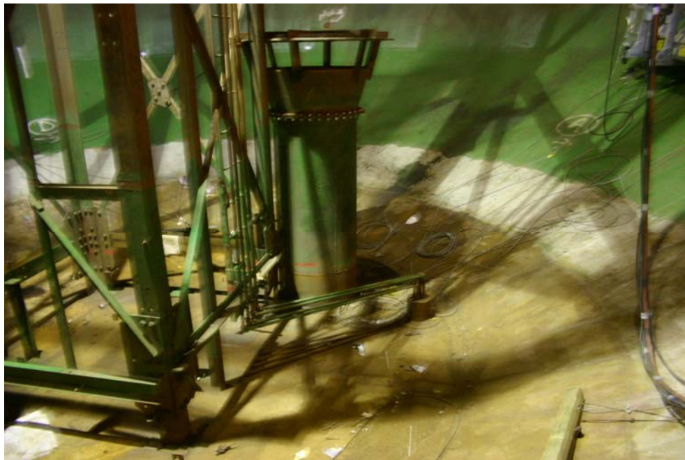
Photograph 12 – Bottom of the tank. Note the 32-inch inlet/outlet line and the 4 x \frac{3}{4} -inch sample lines.
