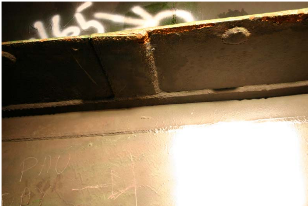
Photograph 10 – Underside of the expansion joint, quadrant A, vertical drop 15.
