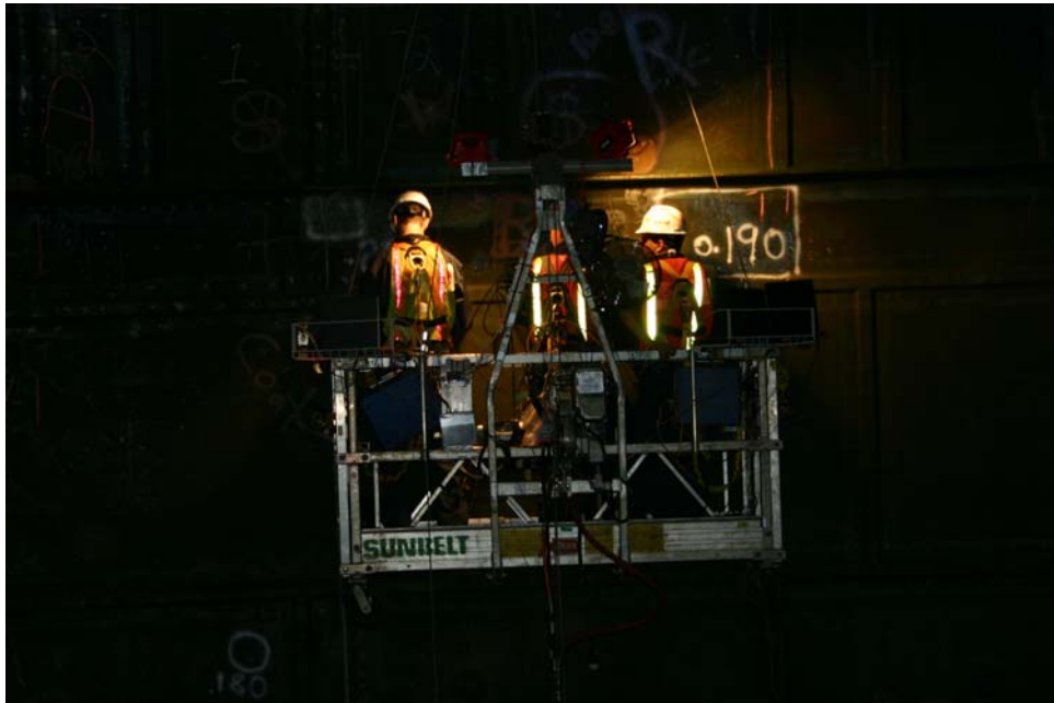
Team one inspecting the extension area of quadrant D.
