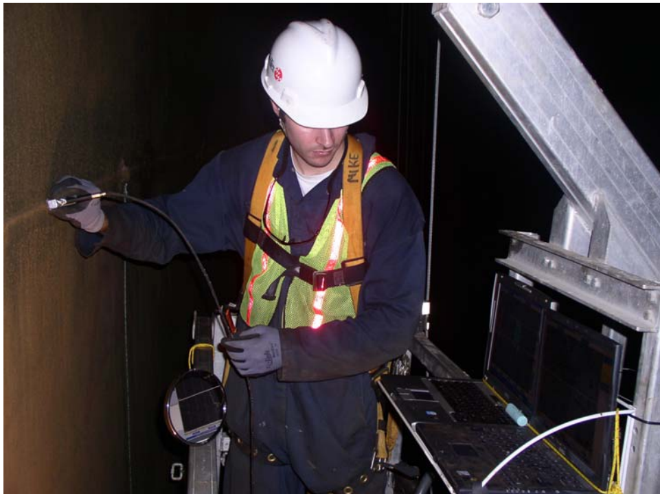
Shows Hawkeye weld scanning under the catwalk.
