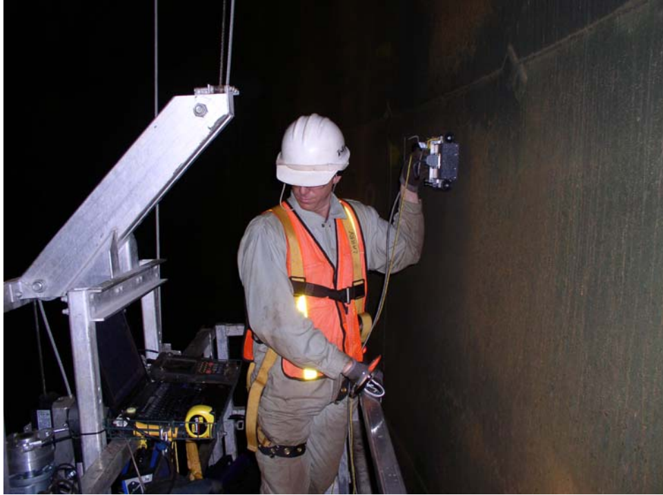
Shows LFET scanning under the catwalk.
