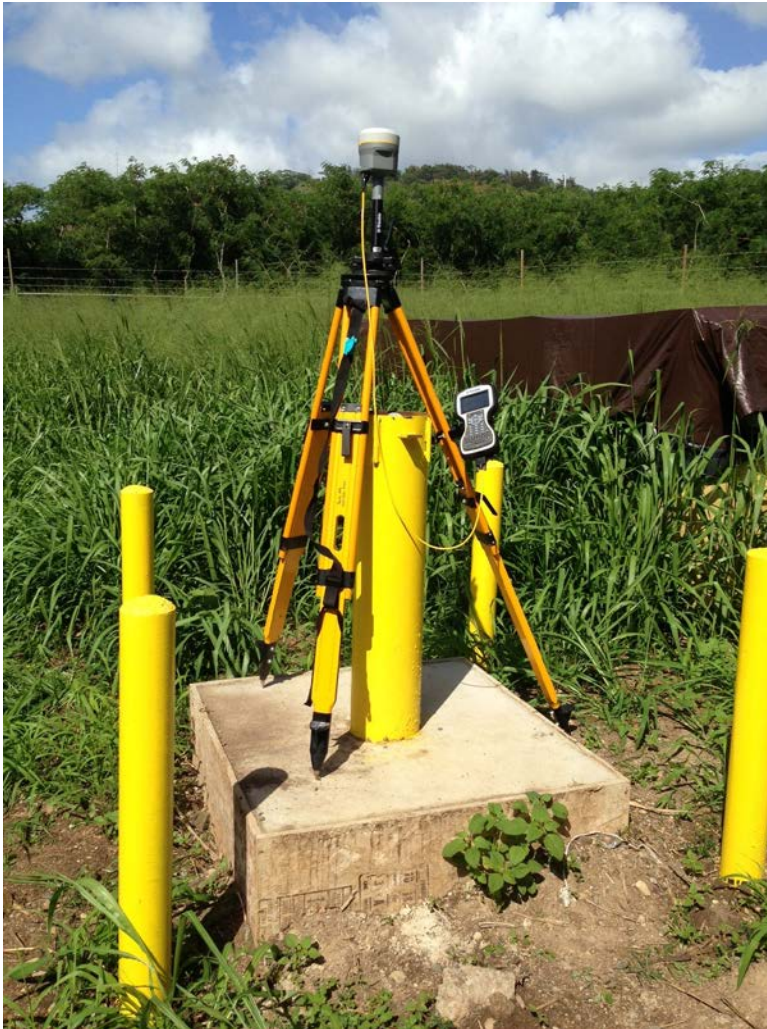
Figure 1. New Monitoring Well
