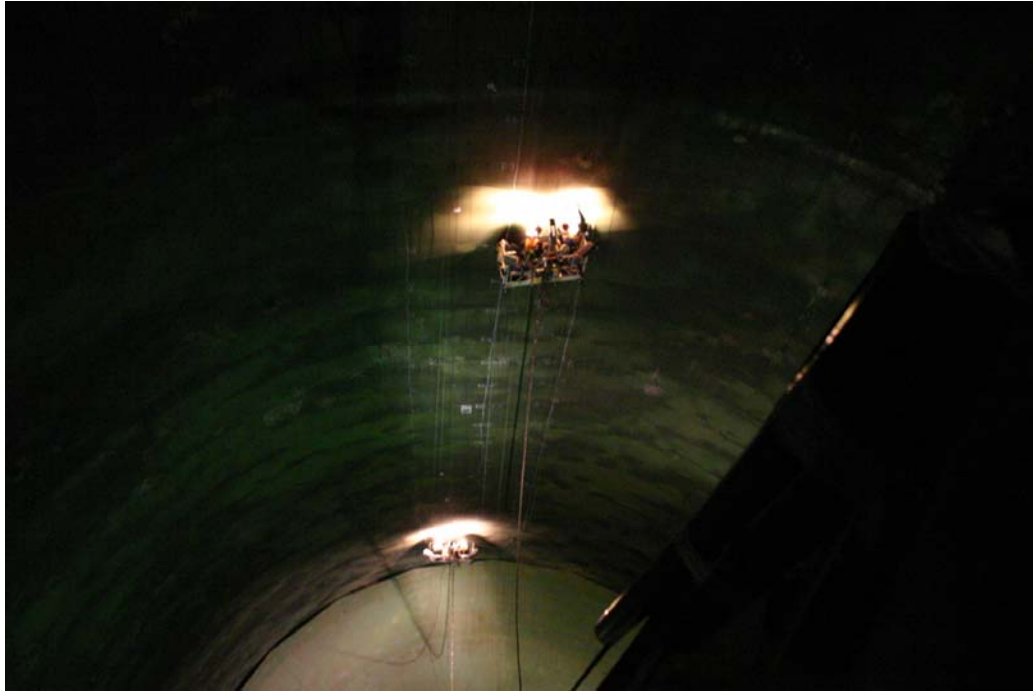
Photograph 3 – A view of the barrel and lower dome from the tower at the catwalk level.
