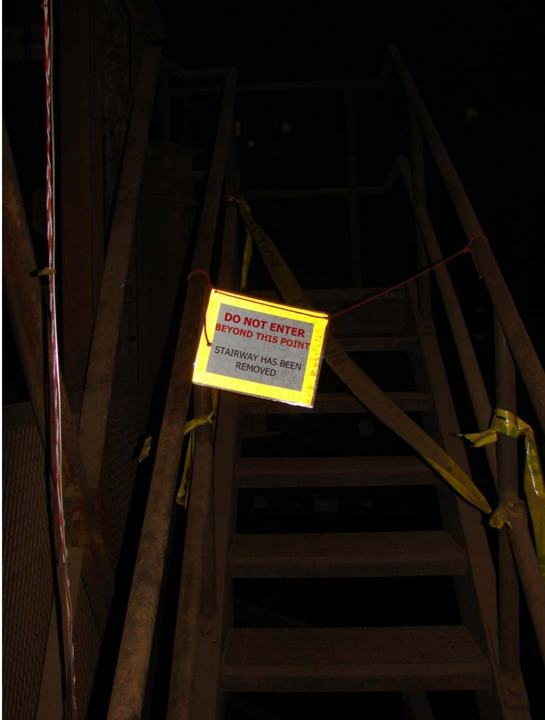
Tower Stair Section Removed & Replaced
