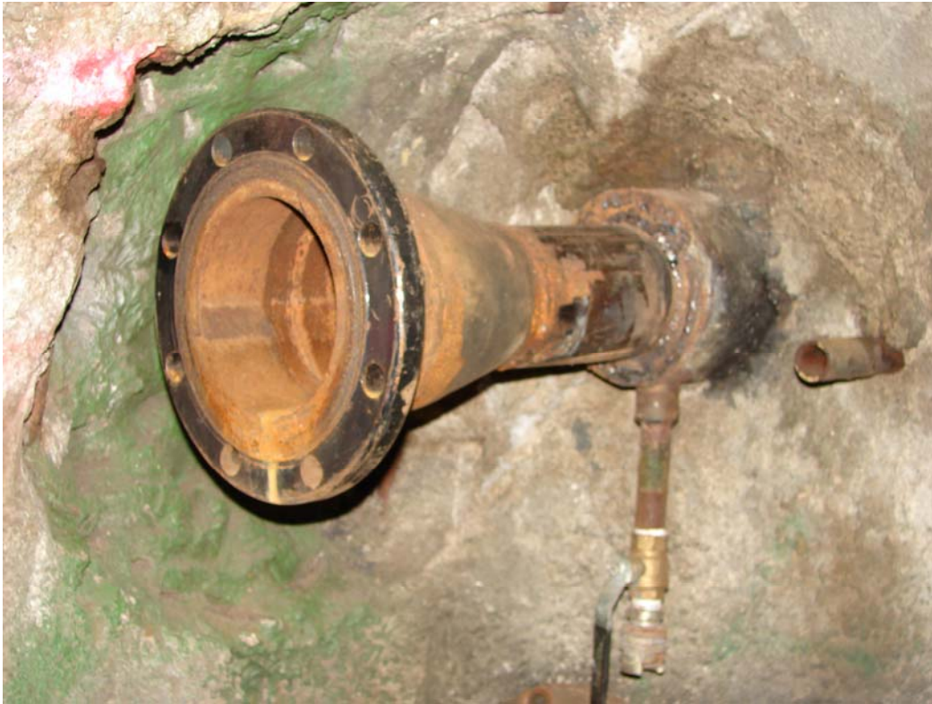
New Slop Line Lower Tunnel
