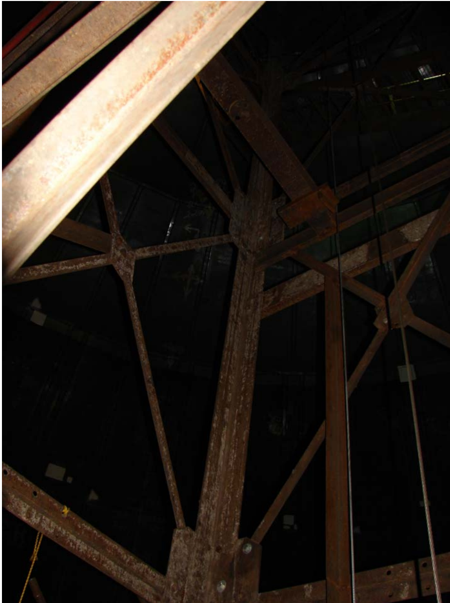
Tower Structural Repairs
