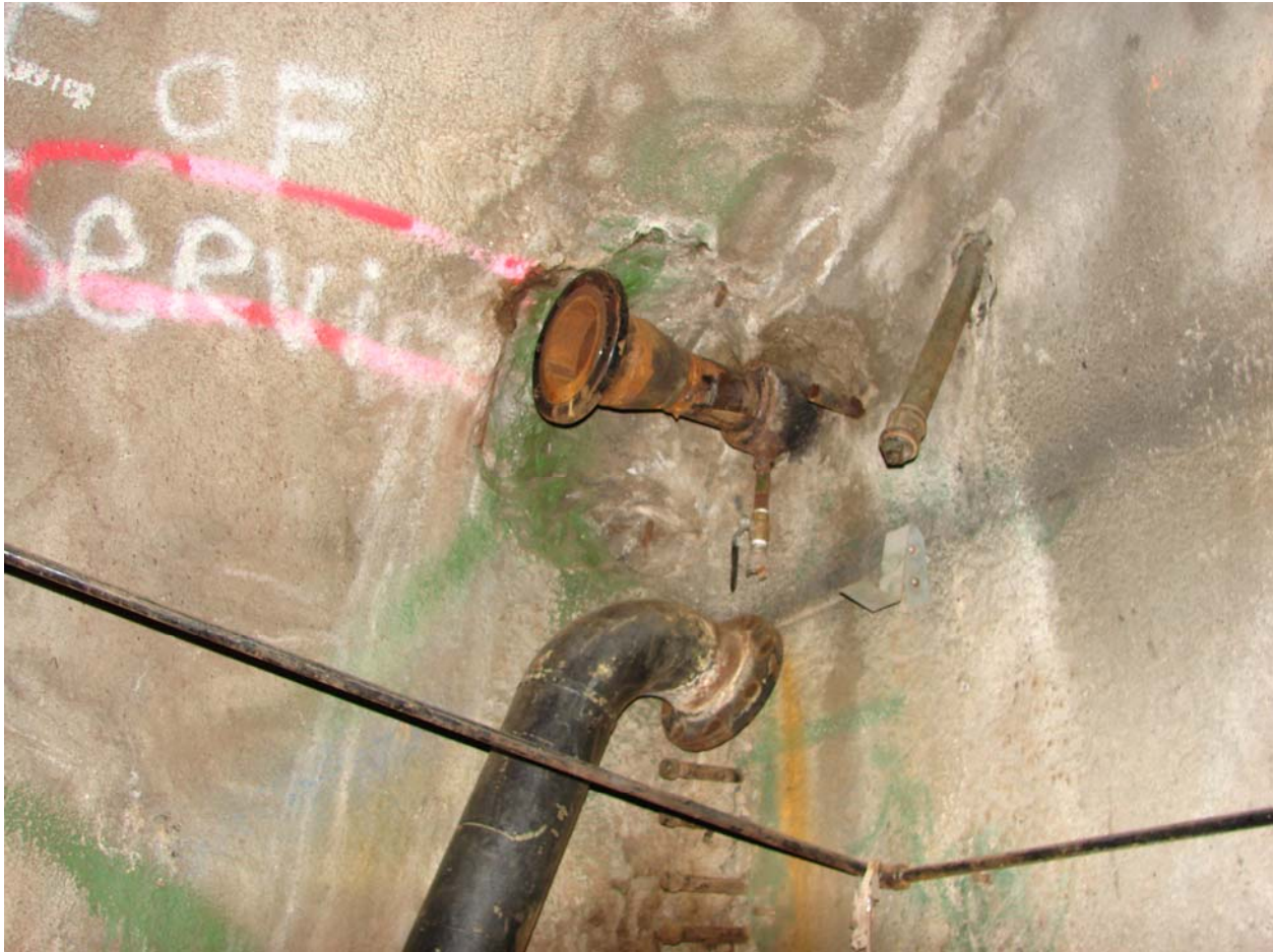
New Slop Line Lower Tunnel
