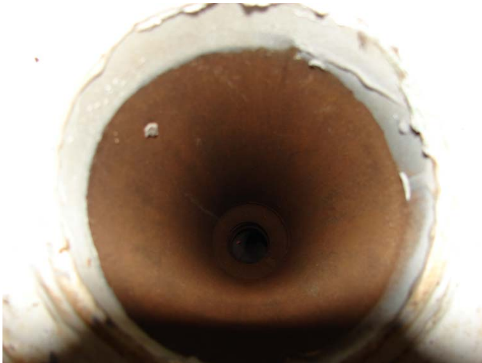
From Inside Tank Looking Down
